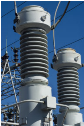
High voltage current Transformer
